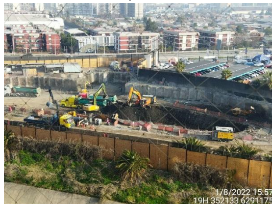
Vista general norte
