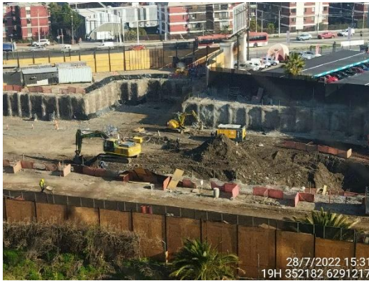
Vista general norte
