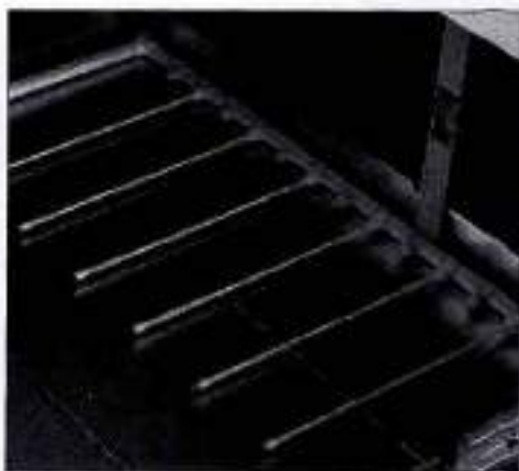
Basin Sweeper Piping
