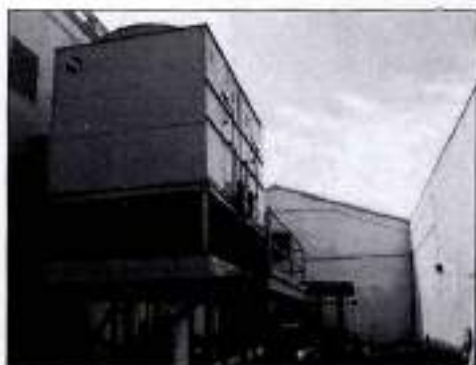
EVERTOUGH™ Construction Installation
