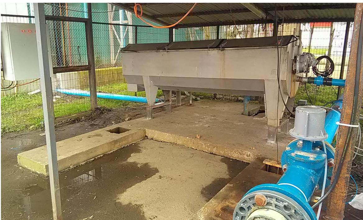
Figura 10: Rotofiltro Rotomaster
