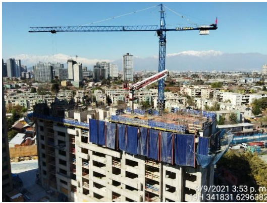
Vista general Torre 8
