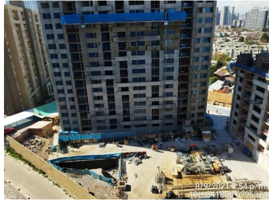
Vista general Torre 9
