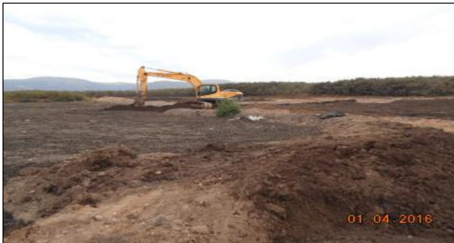
Vaciado piscina sector 3 ( 35^{\circ}12'16.31''S ) ( 71^{\circ}23'6.84''O )
