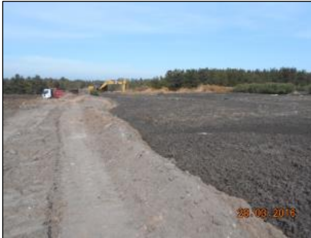
Vaciado piscina sector 3 (35°12'16.31"S) (71°23'6.84"O)
