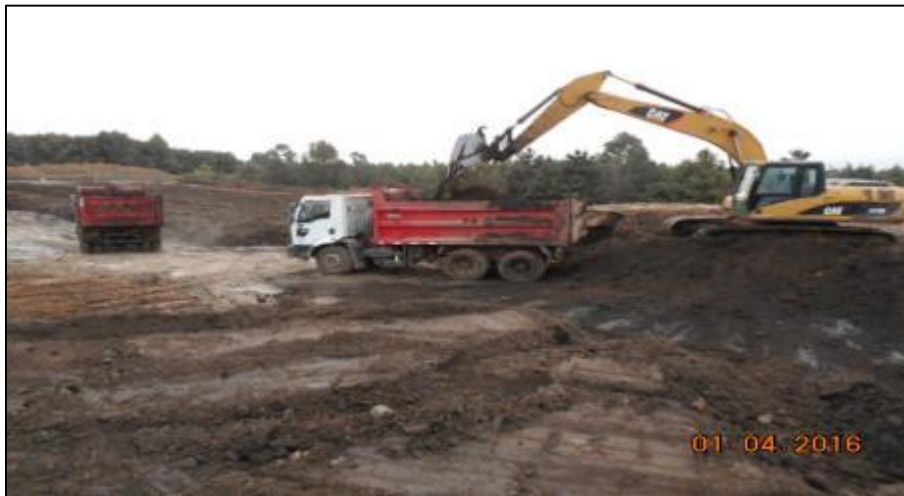
Vaciado de piscina sector 3 ( 35^{\circ}12'16.16''S ) ( 71^{\circ}23'6.54''O )
