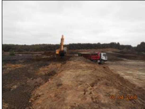
Vaciado de piscina sector 3 ( 35^{\circ}12'16.41''S ) ( 71^{\circ}23'6.92''O )
